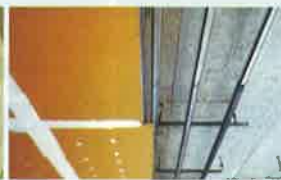
GYPSUM BOARD CEILING
