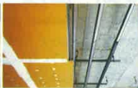
GYPSUM BOARD CEILING
