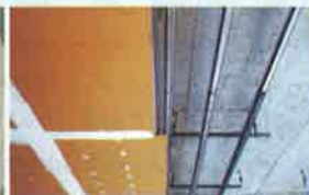
GYPSUM BOARD CEILING
