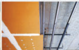
GYPSUM BOARD CEILING
